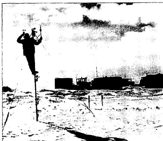
Fig. 1 AWS during installation inland of Mawson. An anemometer, wind vane and temperature sensor are mounted 4 m above the surface with additional temperature sensors at 2 m and 1 m. The transmitter antenna (nearest the guy) and breather pipe for the batteries are downward from the mast.
