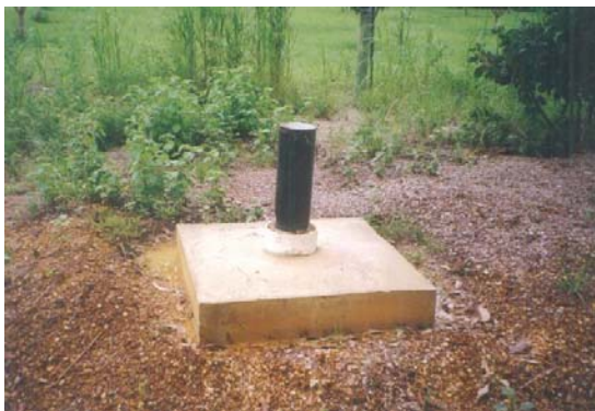
Capped Bore, Darwin Rural Area
