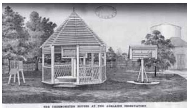
Figure 3. Illustration of instrument comparison at Adelaide, showing a Stevenson screen (left), an octagonal 'thermometer house' (centre) and a Glaisher stand (right).
