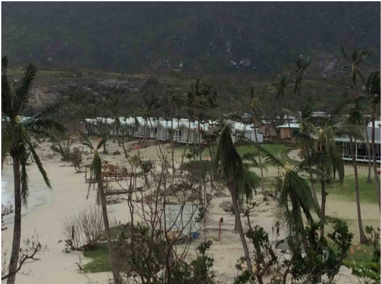
Figure 17. Aftermath of Nathan on Lizard Island. Photo supplied via Queensland Fire and Emergency Services (QFES).
