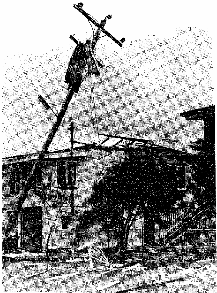
Damaged buildings at Kurrimine beach.
