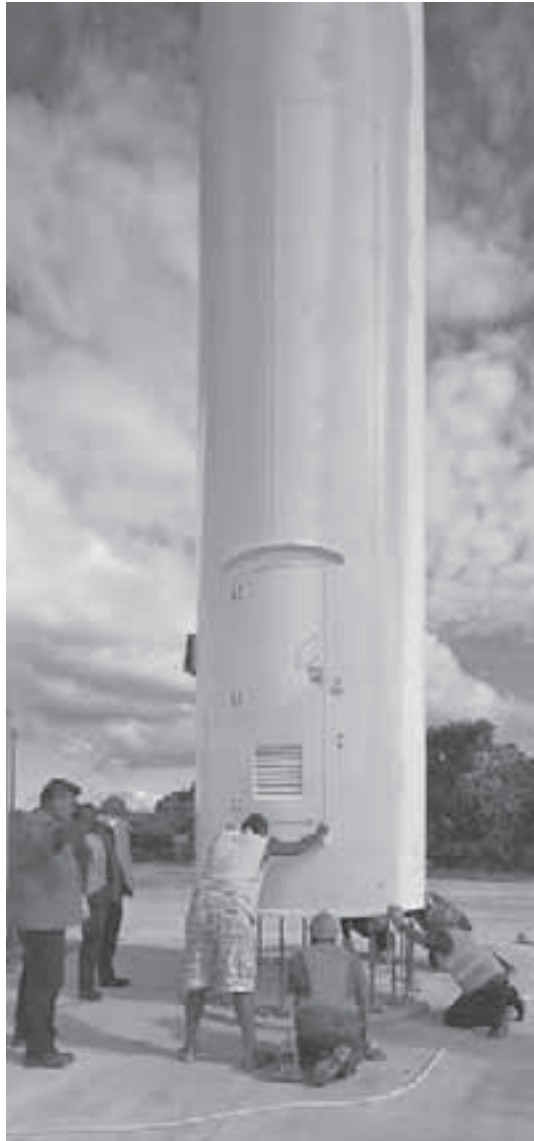
Under the keen eye of Bureau of Meteorology and Meteo France personnel, the first of two 7.5 metre sections of the New Caledonian radar tower is lowered onto its base.
