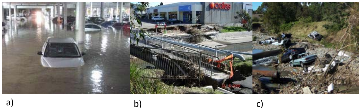
Figure 4 Flood damage (a) supermarket car park, (b) footbridge abutment, (c) car yard debris.
