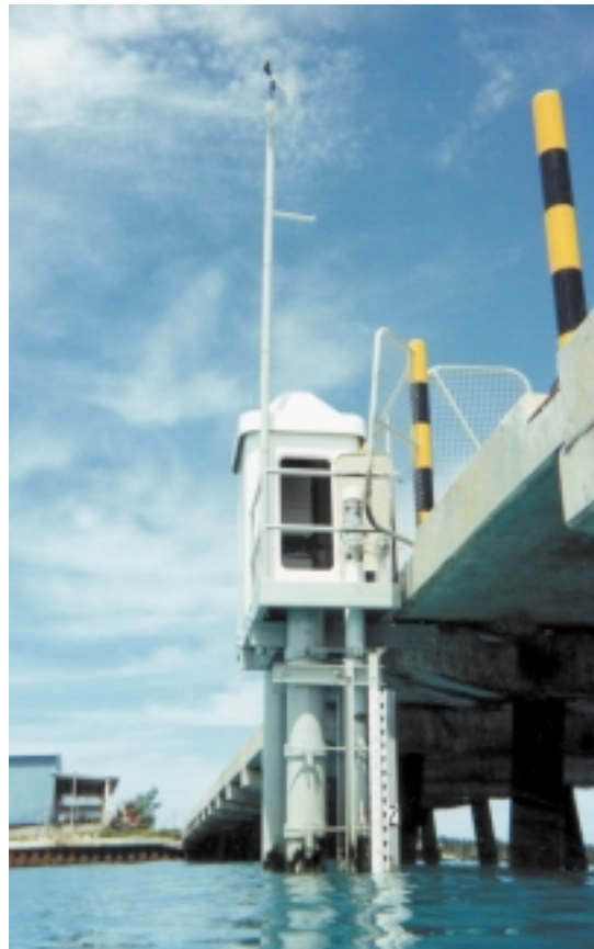
Seaframe Station at Betio, Kiribati.
