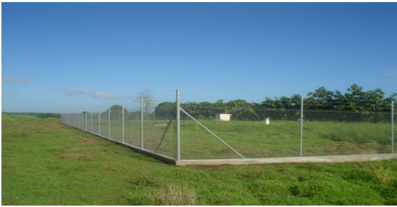
Fencing of CGPS at Faagalii Airport, Samoa.
