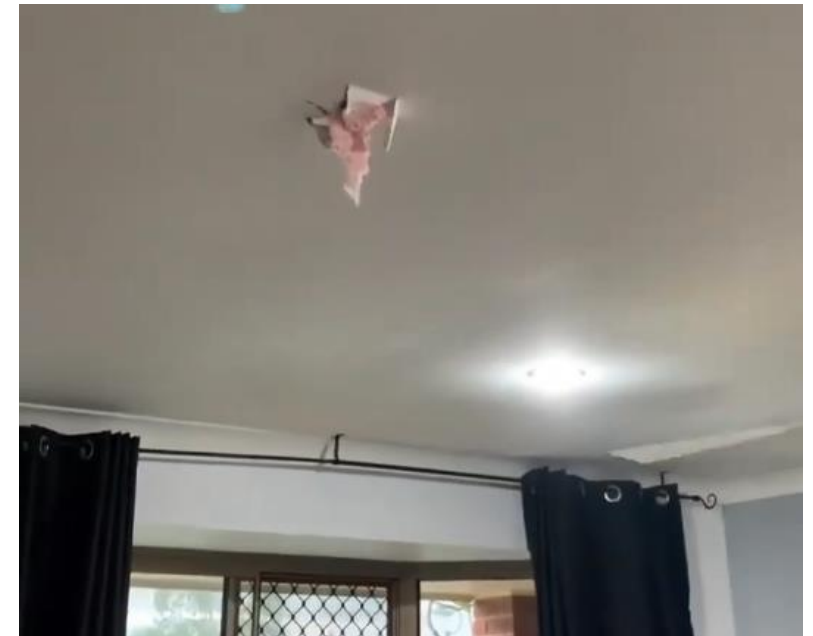
Internal ceiling perforations (ABC Brisbane, 2020)
