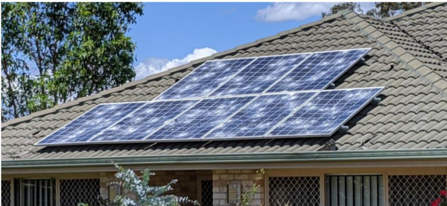
Solar Panel Damage (Wind Research Lab, UQ, 2020)
