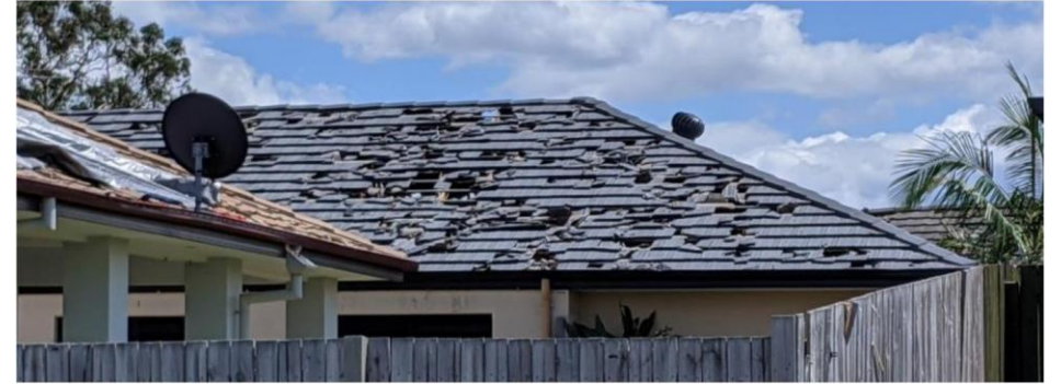
Concrete tile roof damage (Wind Research Lab, UQ, 2020)
