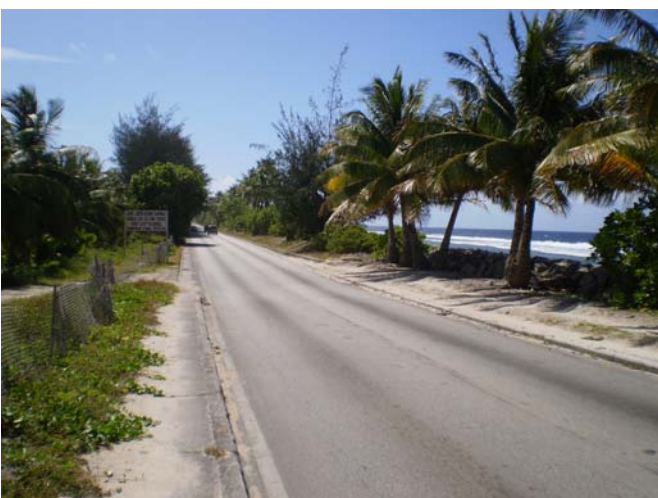
Main road between airport and Majuro with 1 metre raised sea barrier
