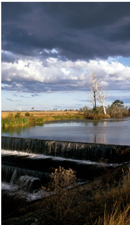
Weir on Barambah Creek near Murgon, S.E. Queensland. (Image credit: Brad Sherman, CSIRO)
