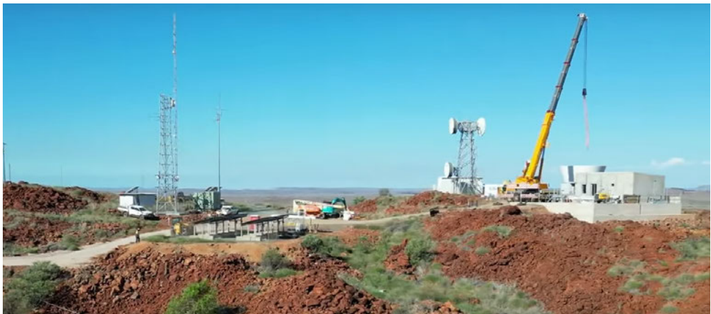
Construction of the new Karratha radar.
