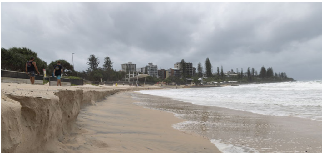
Beach erosion at Kings Beach in Caloundra caused by tropical cyclone Alfred.
