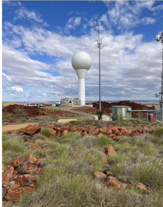
The new Karratha radar was installed in October.
