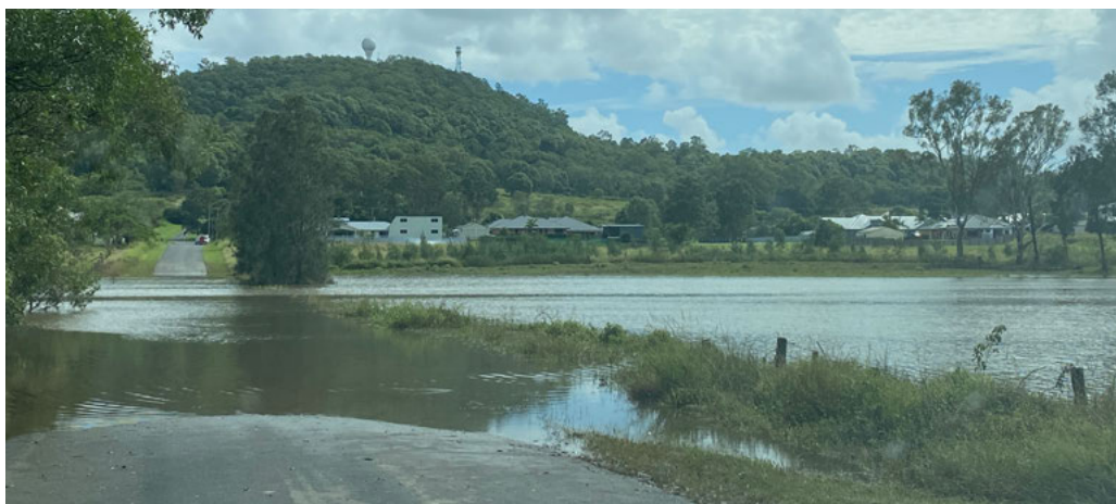
Flooding closed the road to the Mt Stapylton radar following tropical cyclone Alfred in March.
