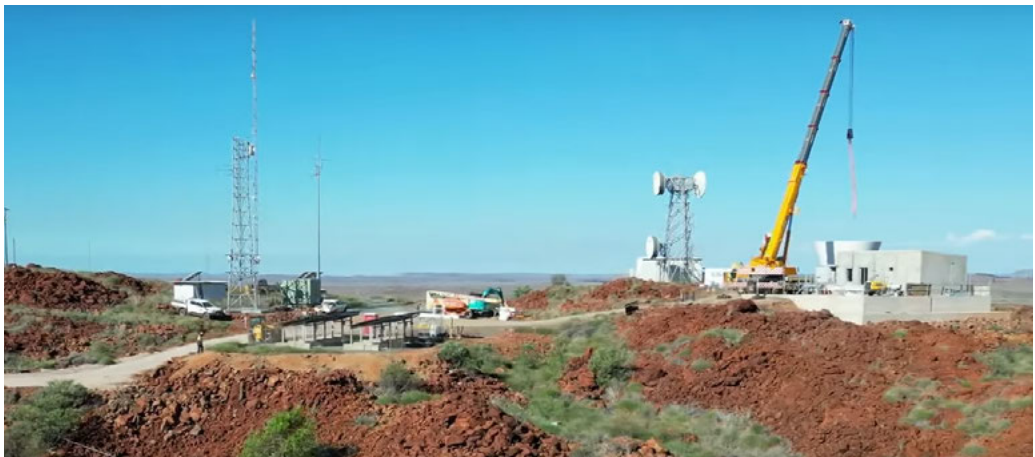
Construction of the new Karratha radar.
